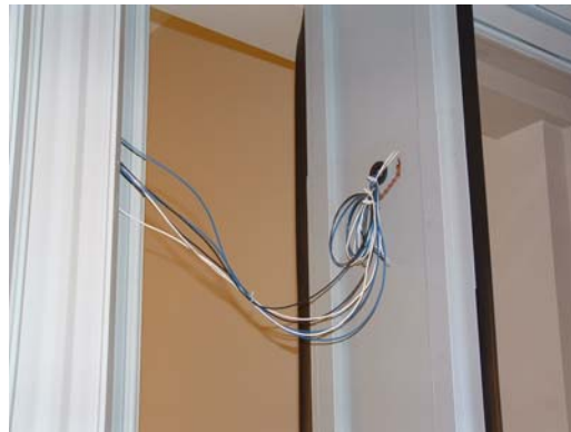
Figure 12b. Leaving Extra Wiring
