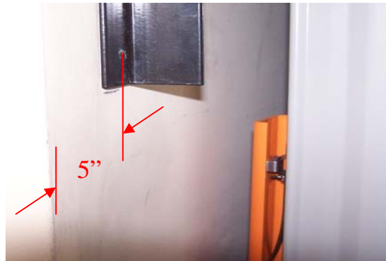
Figure 15. Jamb Stop and Exit Hardware
