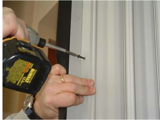
Figure 11. Attaching Jamb Section to Floating Jamb
