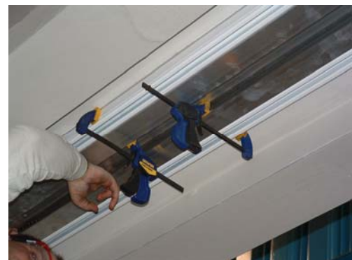
Figure 3.5b. Using Clamps to Secure Chain
