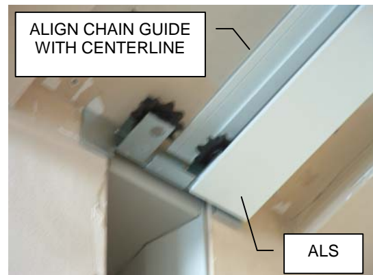
Figure 3.1. Chain Guide Loading Section and Sprocket Assembly
