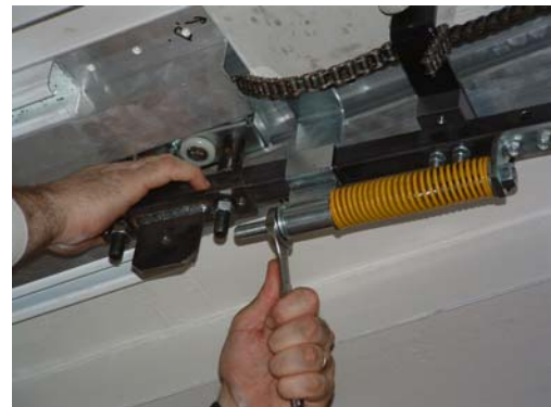
Figure 3.6. Adjusting Chain Tension
