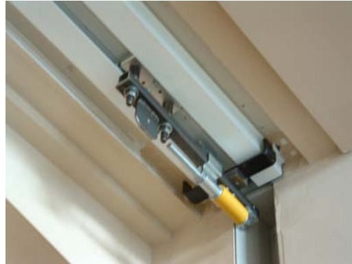
Figure 6.1. Trolley in Position for Loading Curtain (Straight Track Configuration shown)
