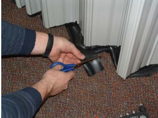
Figure 13a. Trimming Sweep from Outside
