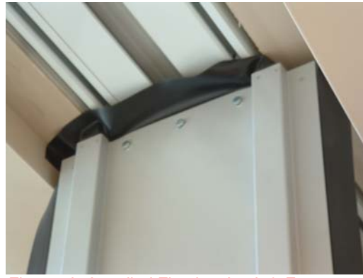
Figure 7b. Installed Floating Jamb & Fasteners
