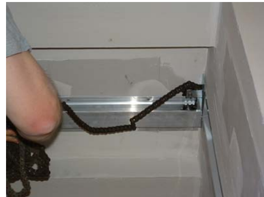
Figure 3.5a. “Threading” End Sprocket Assembly
