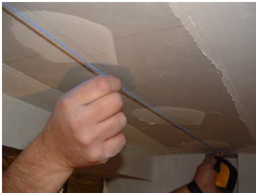
Figure III.1. Marking the Centerline
